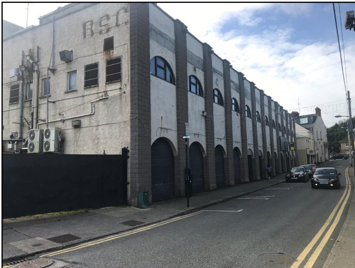
Figure 3.1 – View from Quay Street of former Mall Shopping Centre (to be demolished)
