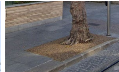
Urban tree pit with permeable resin bound gravel tree surrounds are proposed to hug the kerb on High Street, maximising space for pedestrians. Example Dawson Street, Dublin City Centre
