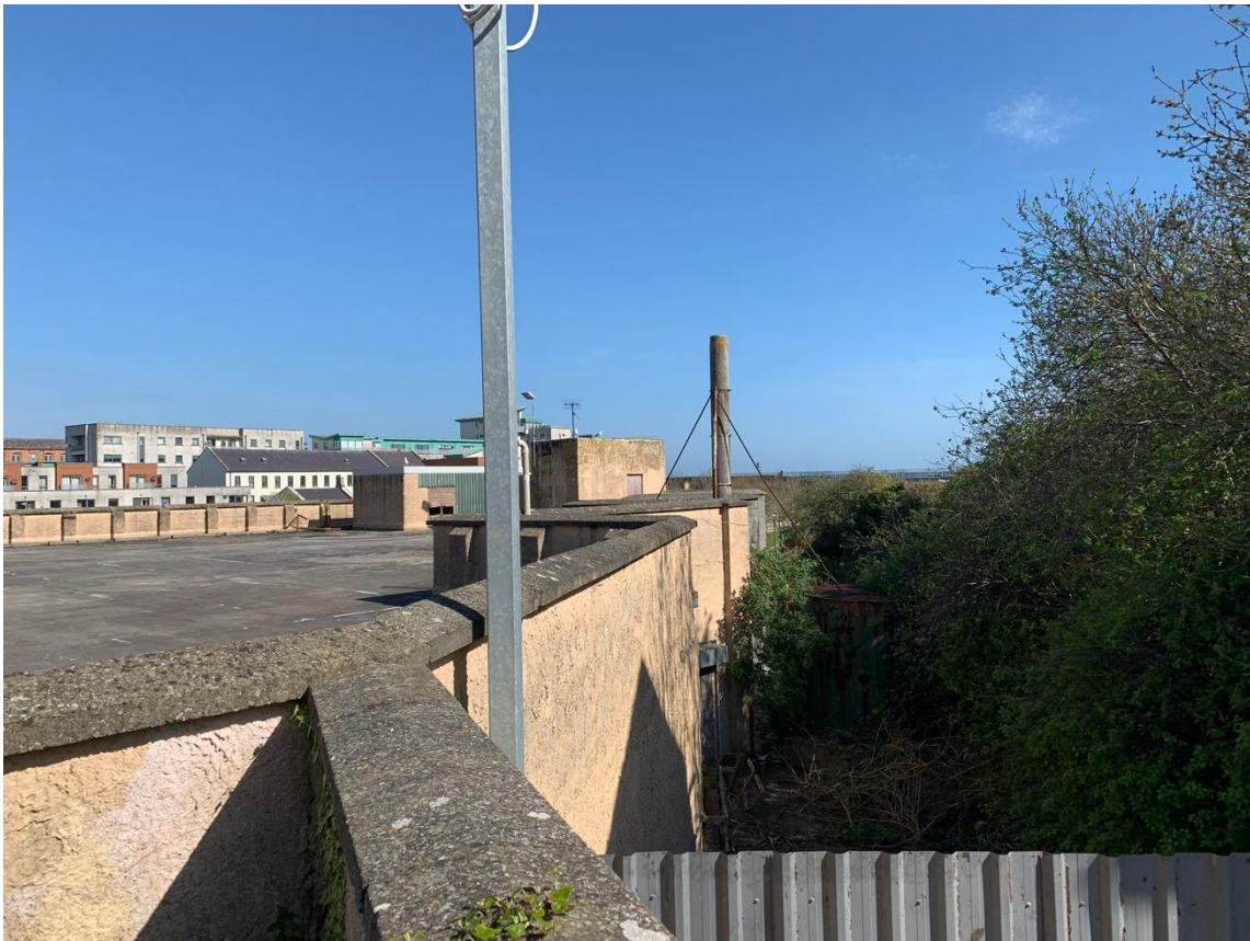
Plate 20 The existing boundary condition at the rear of the High Street properties. A new concrete retaining wall will be constructed; approximately aligned with this existing boundary.
