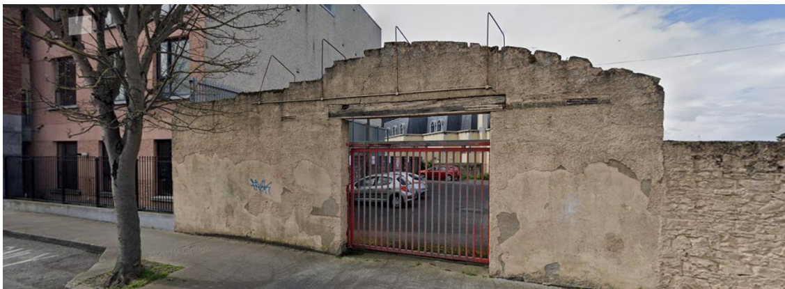
Plate 14 The boundary on High Street is partially comprised of the surviving façade of a wide span building, constructed in the 1930's. The profile of the agricultural-style barrel-vault roof is visible in the façade. This wall is not considered to be of particular architectural interest.
