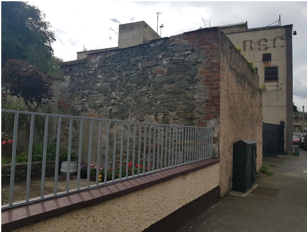
Plate 17 The east side of the northern boundary wall facing onto Quay Street incorporates fabric from an earlier building. It is proposed to retain this fragment in part and incorporate it into the proposed scheme.
