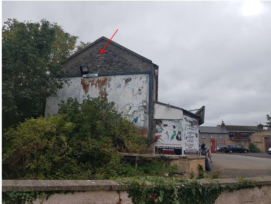
Plate 19 Note the modification to the existing vernacular building. The profile of the gable has been raised and the pitch altered to accommodate a new roof structure.
