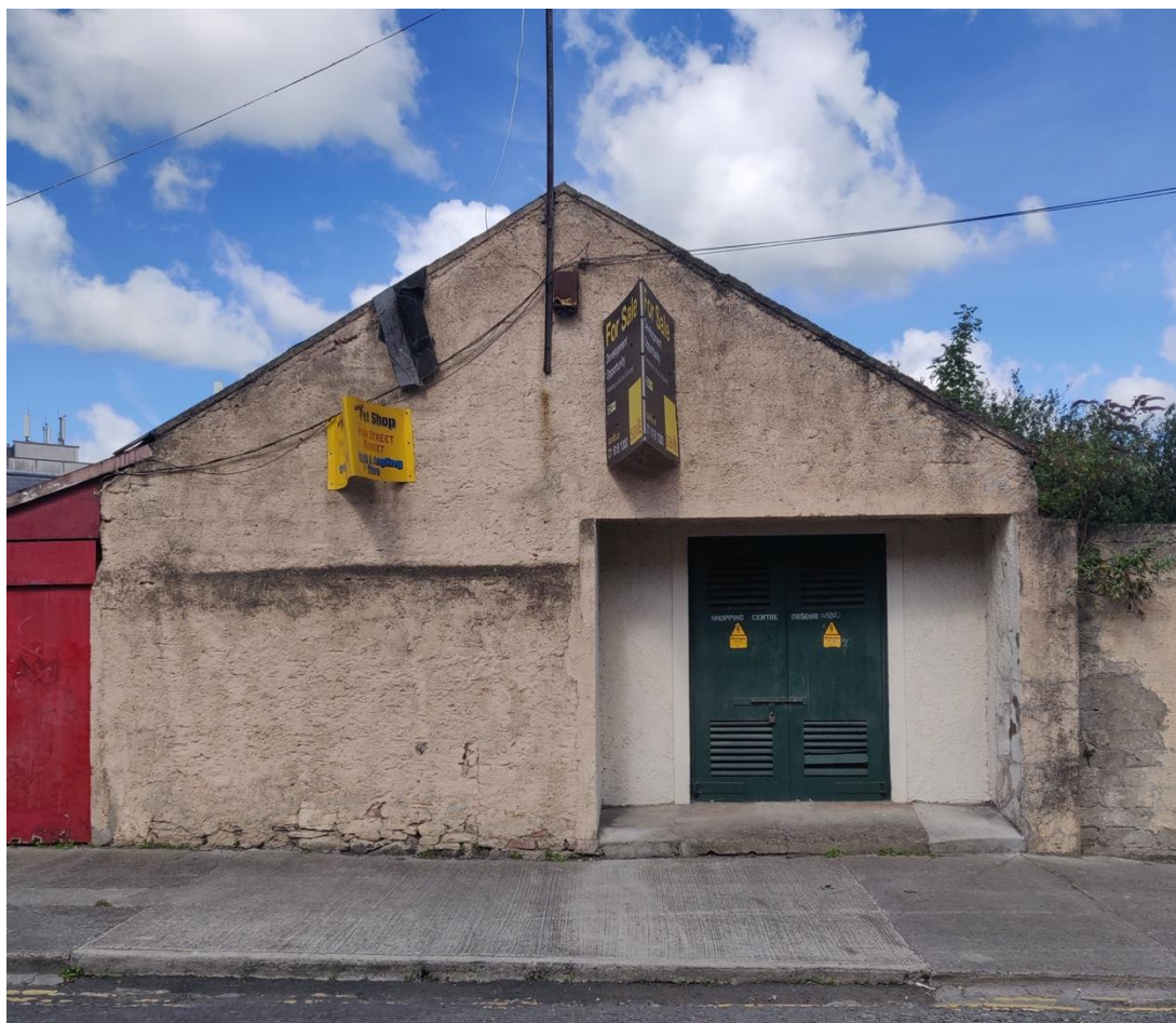
Plate 13 The gable fronted outbuilding, dating from the early 20 th century, fronting onto High Street has been modified to accommodate a substation to serve the former supermarket building.
