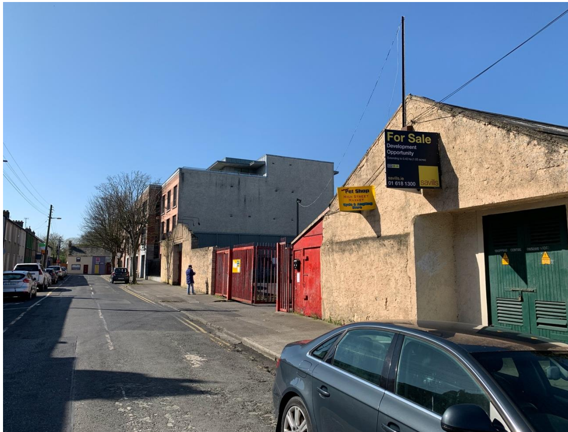
Plate 16 The existing boundary wall on High Street, from south to north (left to right) comprises; a mid 20 th century façade, a length of rubble wall (painted), a wide gated entrance and the gable of an early 20 th century outbuilding modified to house an ESB substation.
